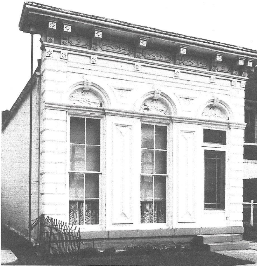
Metal front house in Madison, Ind., one of the first towns in the Trust's Main Street program.
